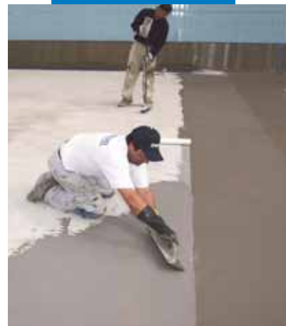
Hydroizolace bazénu Mapelasticem
